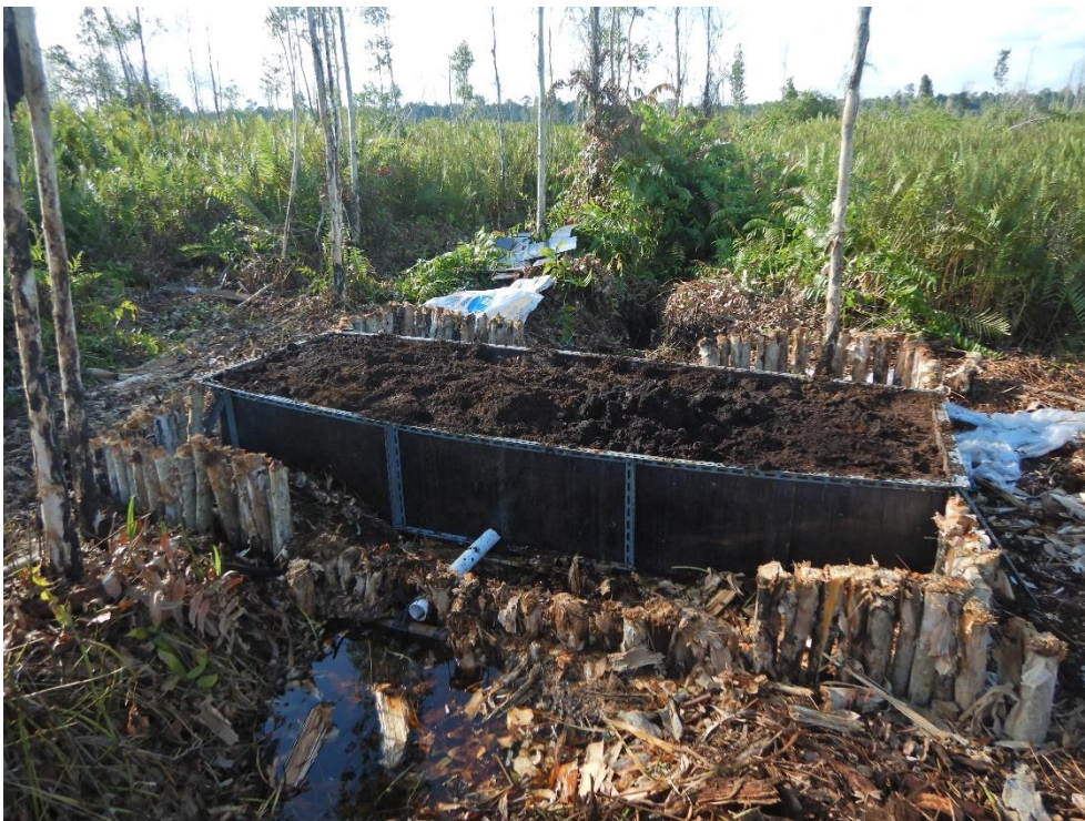
Figure 5. The project team piloting a dam designed on a small former “logging” canal
