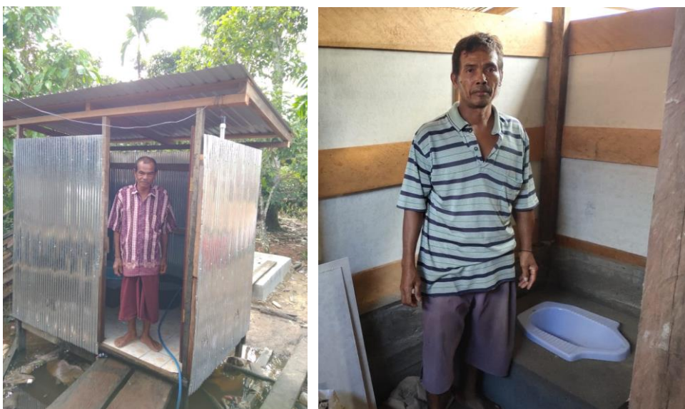
Figure 9. New sanitary latrines in Mendawai village
